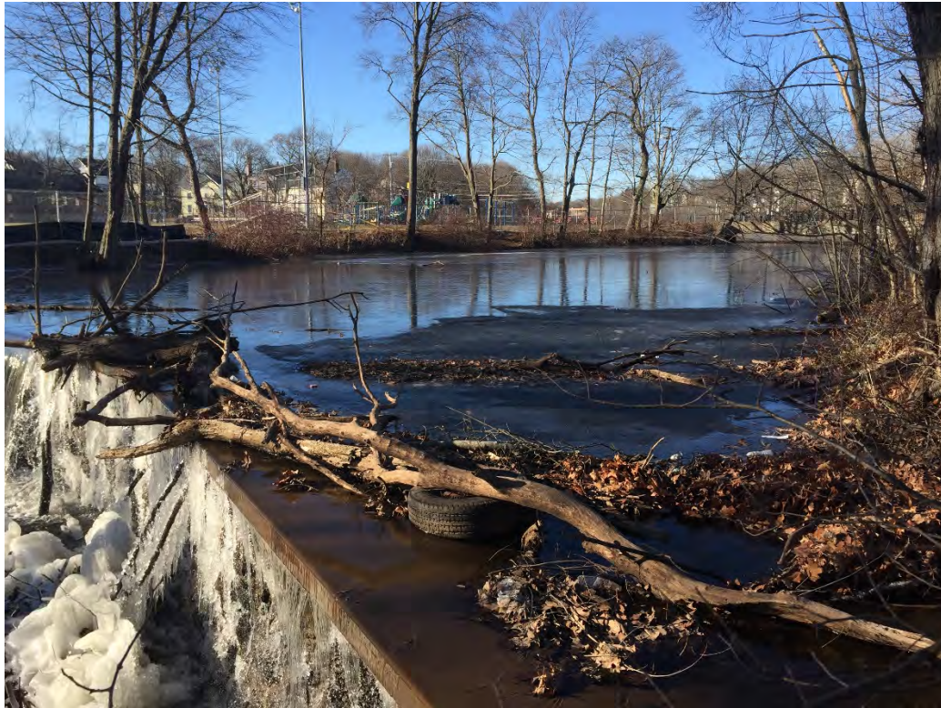
Photo No. 13 – Looking upstream from left abutment.
