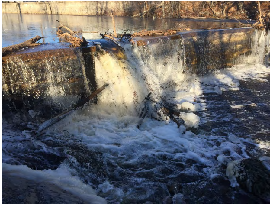
Photo No. 3 – Downstream face and notch (sluiceway).
