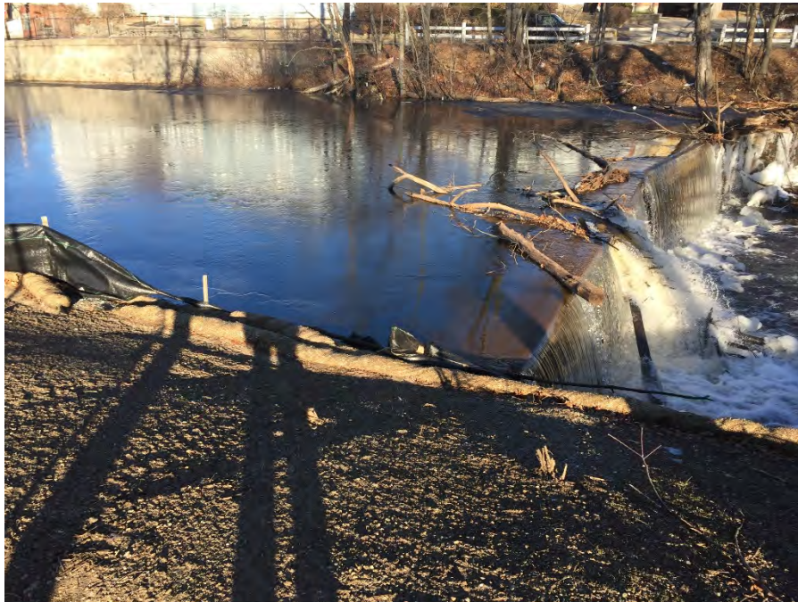
Photo No. 1 – Dam and impoundment viewed from right abutment.
