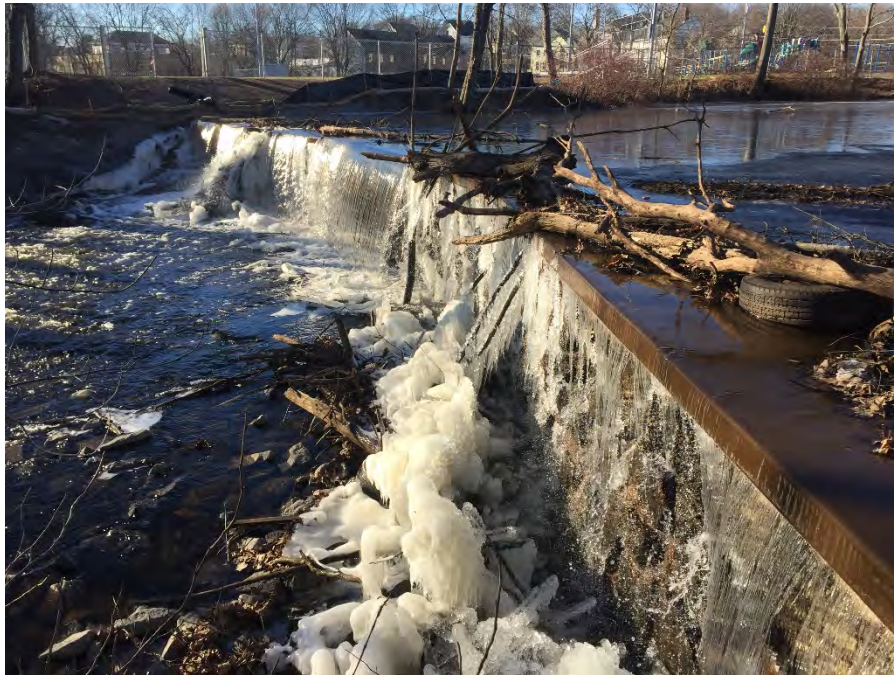
Photo No. 15 – Downstream face, view from left abutment.
