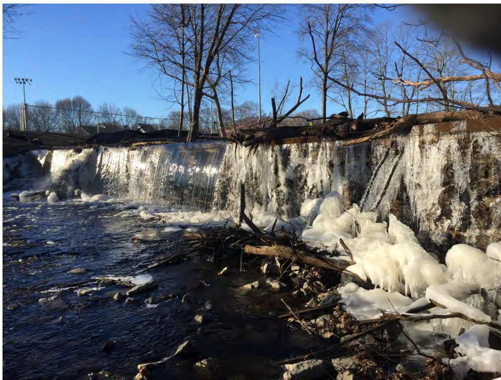
Photo No. 18 – Downstream toe and face from left side.
