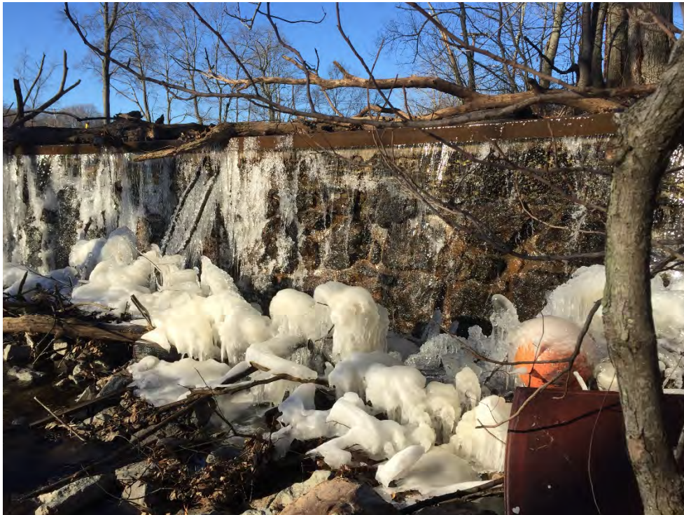
Photo No. 17 – Downstream face view from left downstream toe.
