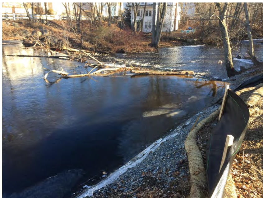
Photo No. 8 – View of impoundment and crest from right bank.
