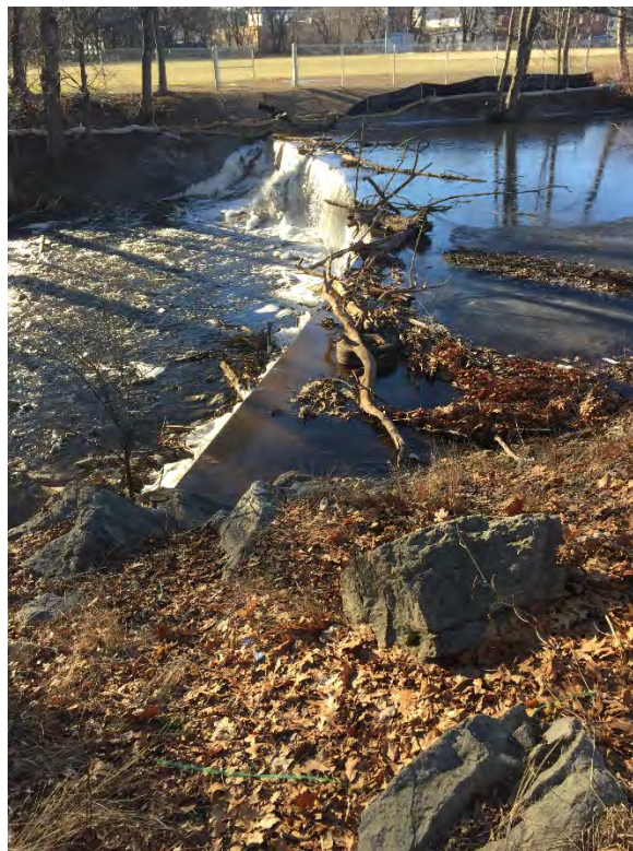
Photo No. 12 – View along crest from left abutment.
