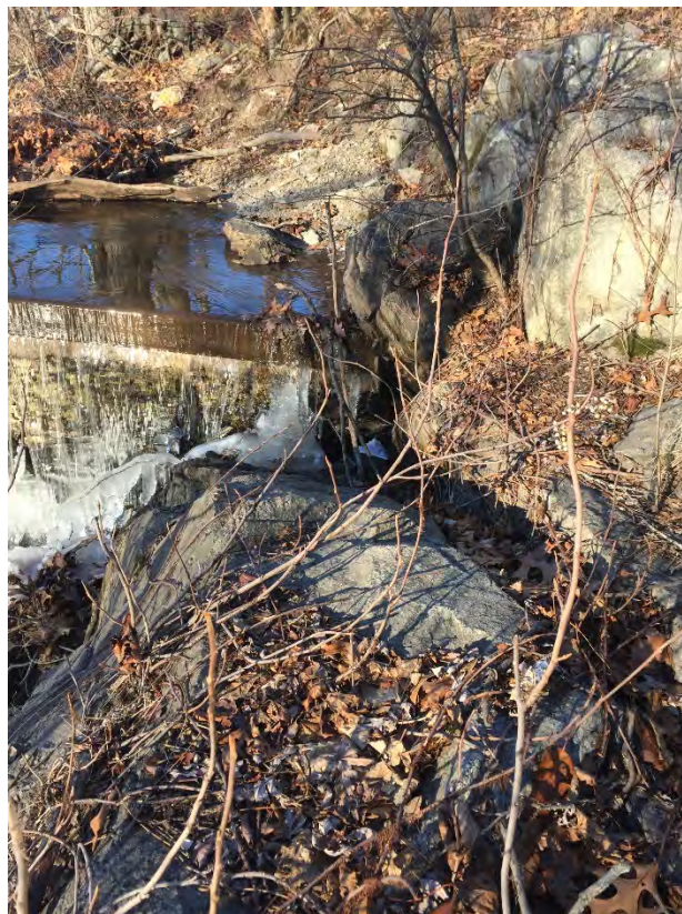
Photo No. 16 – Left abutment interface with bedrock. Note small brush.
