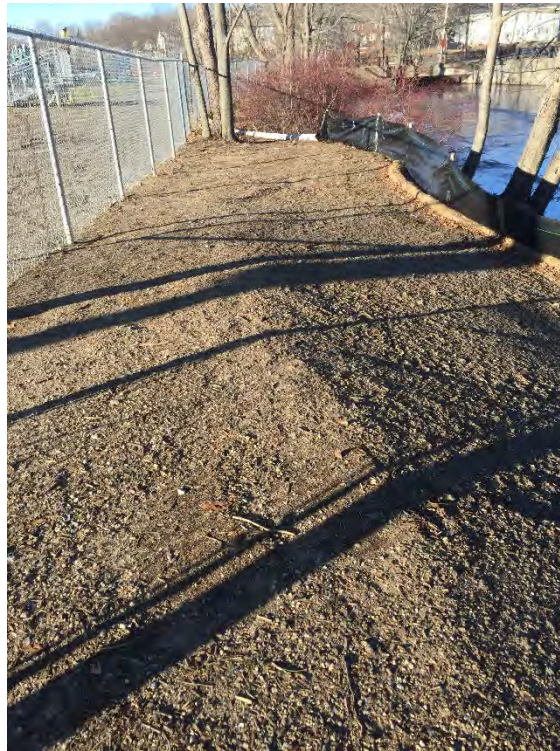
Photo No. 9 – Bank adjacent to right abutment.
