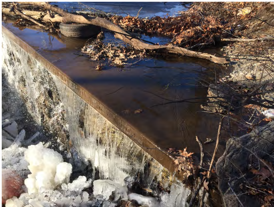
Photo No. 14 – Crest at left abutment.
