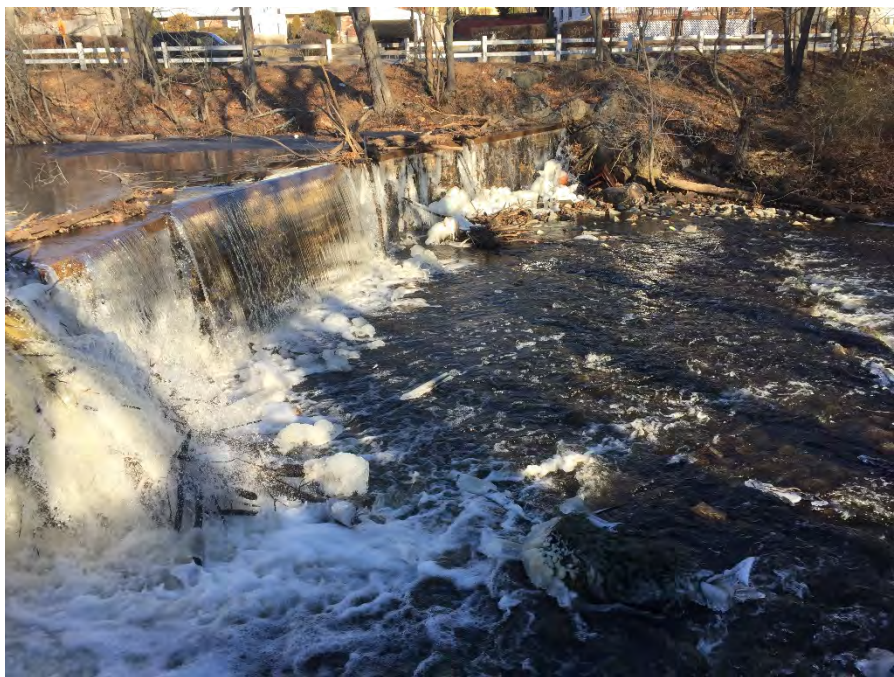
Photo No. 4 – Downstream toe area.
