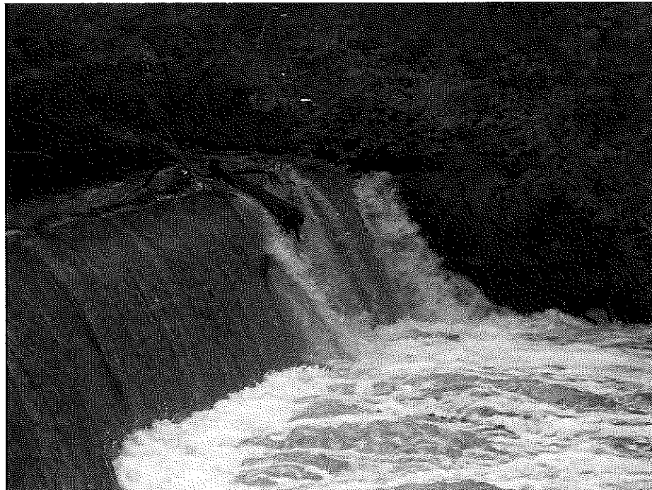
Photo 2 - Left abutment of the dam. Note bedrock abutment and debris.
