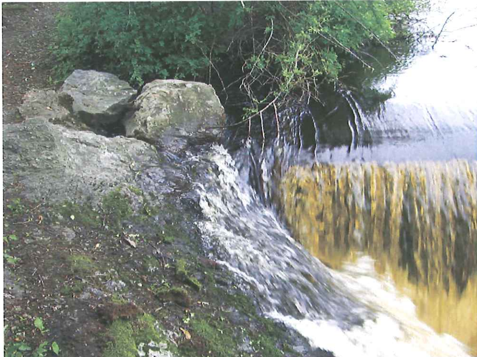
Photo 3 - Right abutment looking upstream. Bedrock abutment at high flow.
