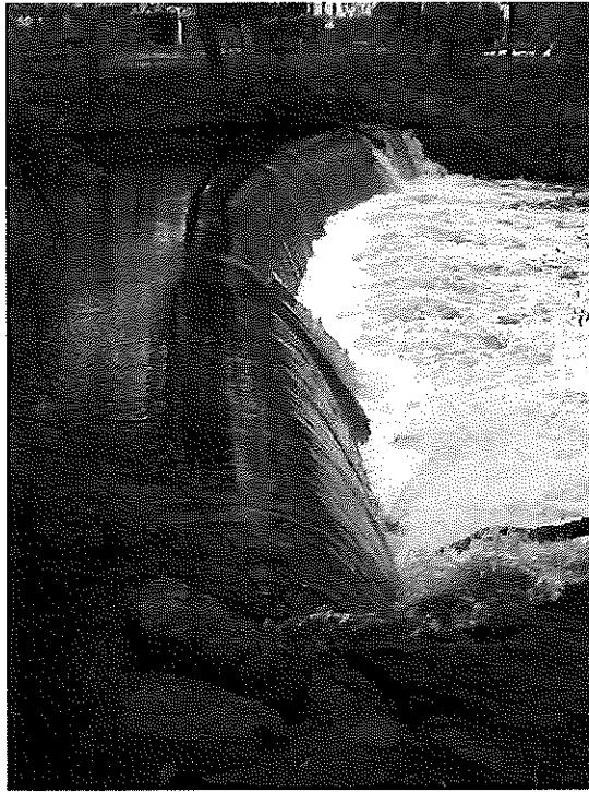
Photo 1 - Colburn Street Dam from the right abutment. Note bedrock abutments, debris on weir, notch or sluice in weir at location of darkened flow.
