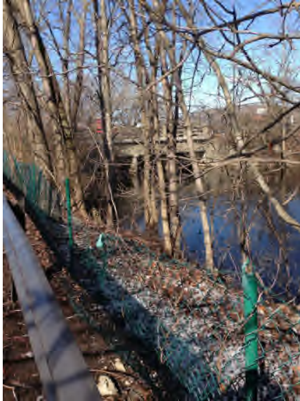
Photograph 1. View upstream of Mother Brook facing Incinerator Road crossing.
