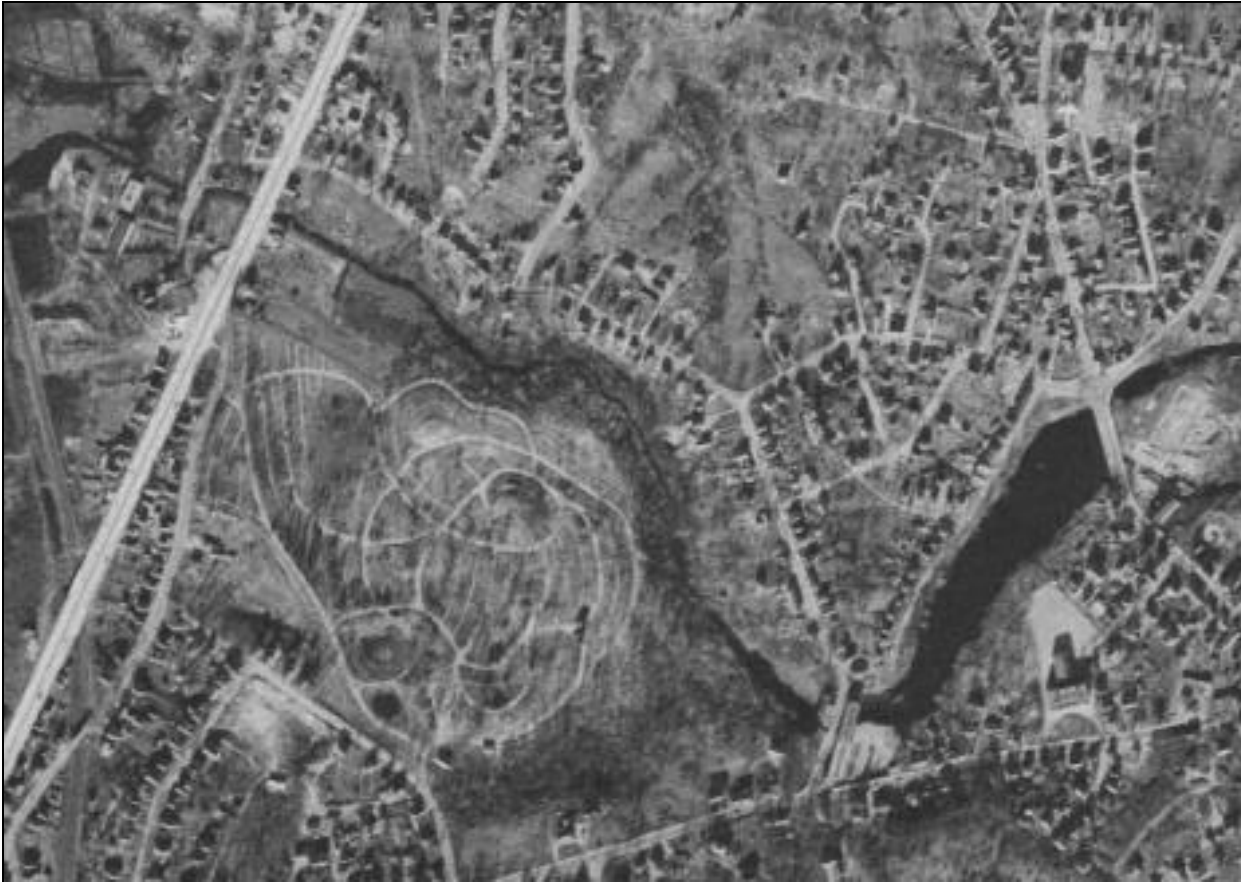
Figure 3. Aerial photograph from 1938 showing Mother Brook prior to rechannelization.
