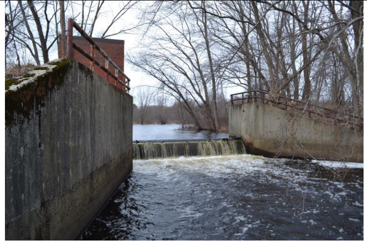
Photograph 2. The Charles River Diversion structure, view west.
