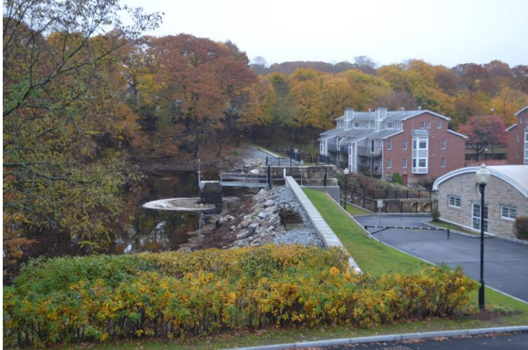
Photograph 13. Centennial Dam at Fourth Privilege, view southeast.
