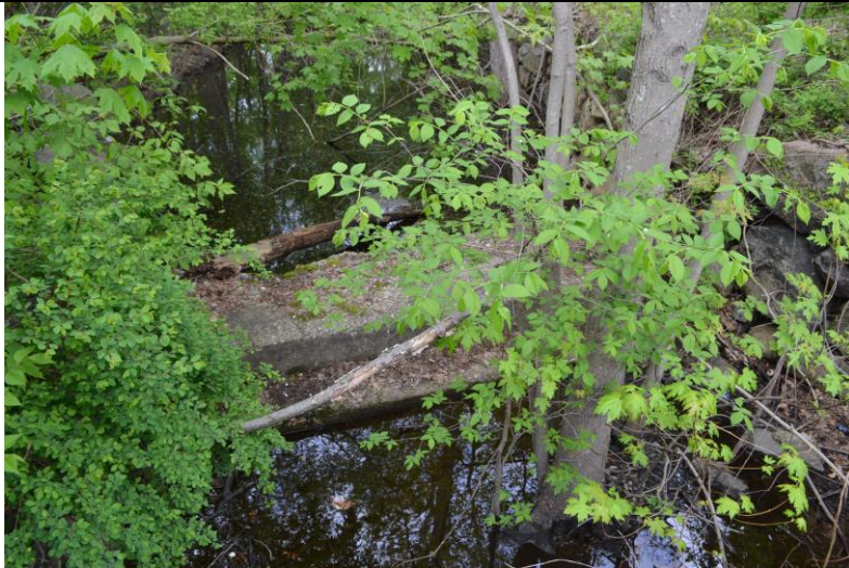
Photograph 5. Dam at Maverick Street, view west.
