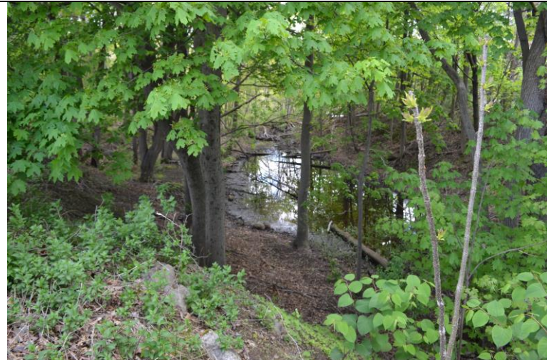
Photograph 8. Overflow spillway at Bussey Street, view southeast.
