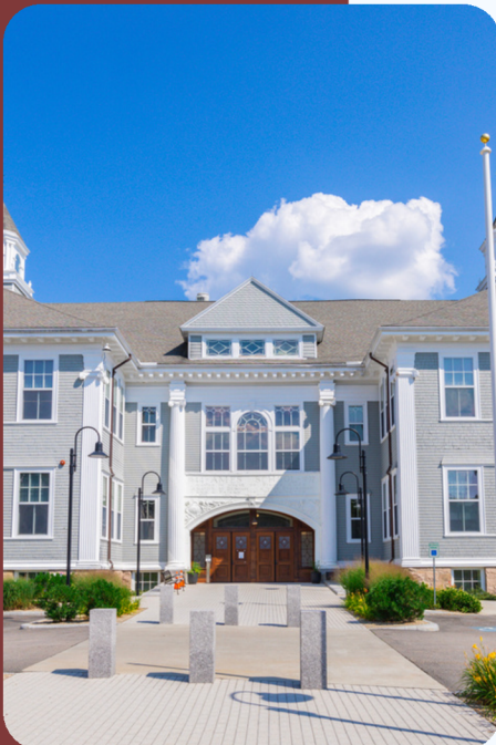
Front entrance to Town Hall
