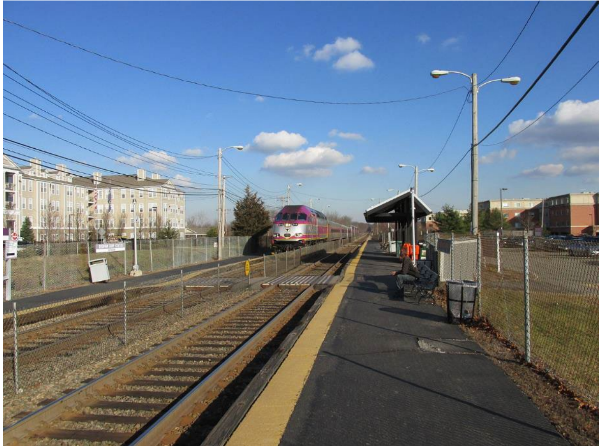
Existing multi-family housing can be seen from the Dedham Corporate Center commuter rail platform.
