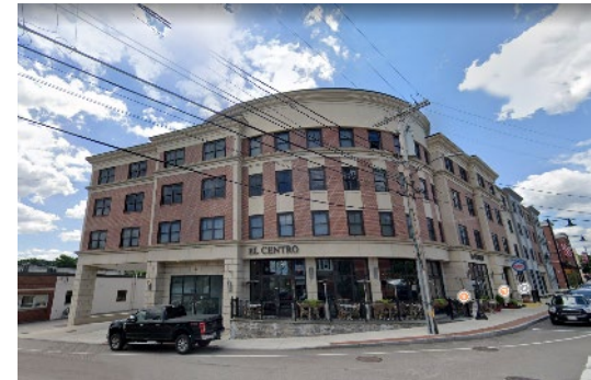
337 Washington St In Dedham Center 107 units/acre
