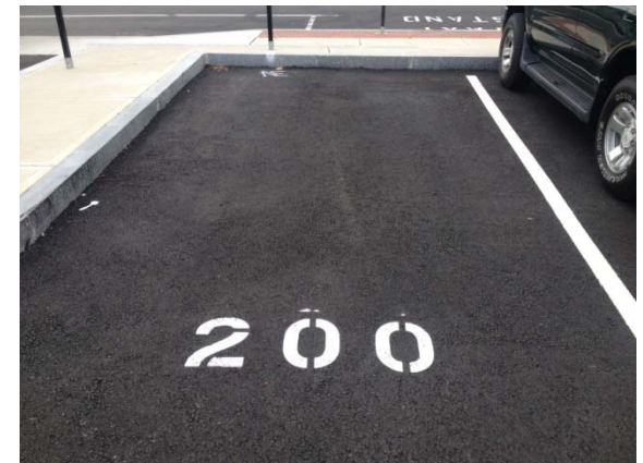
Stall (space) number painted at the top of the stall.
