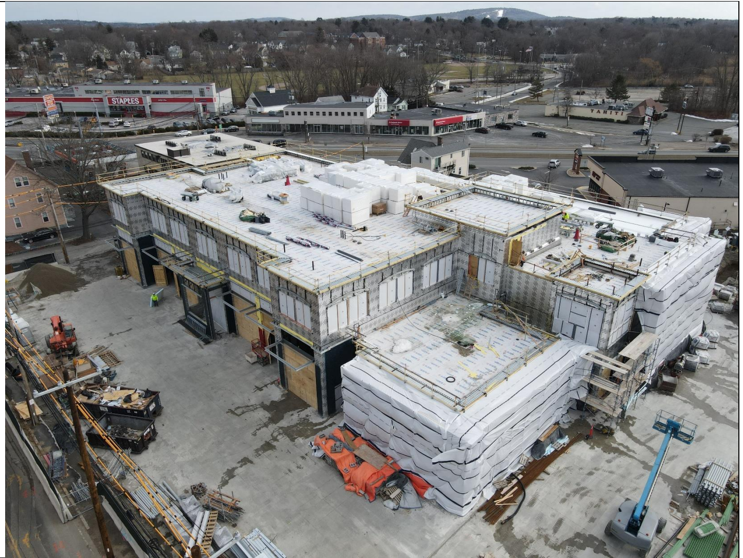
West Elevation Air Barrier System
