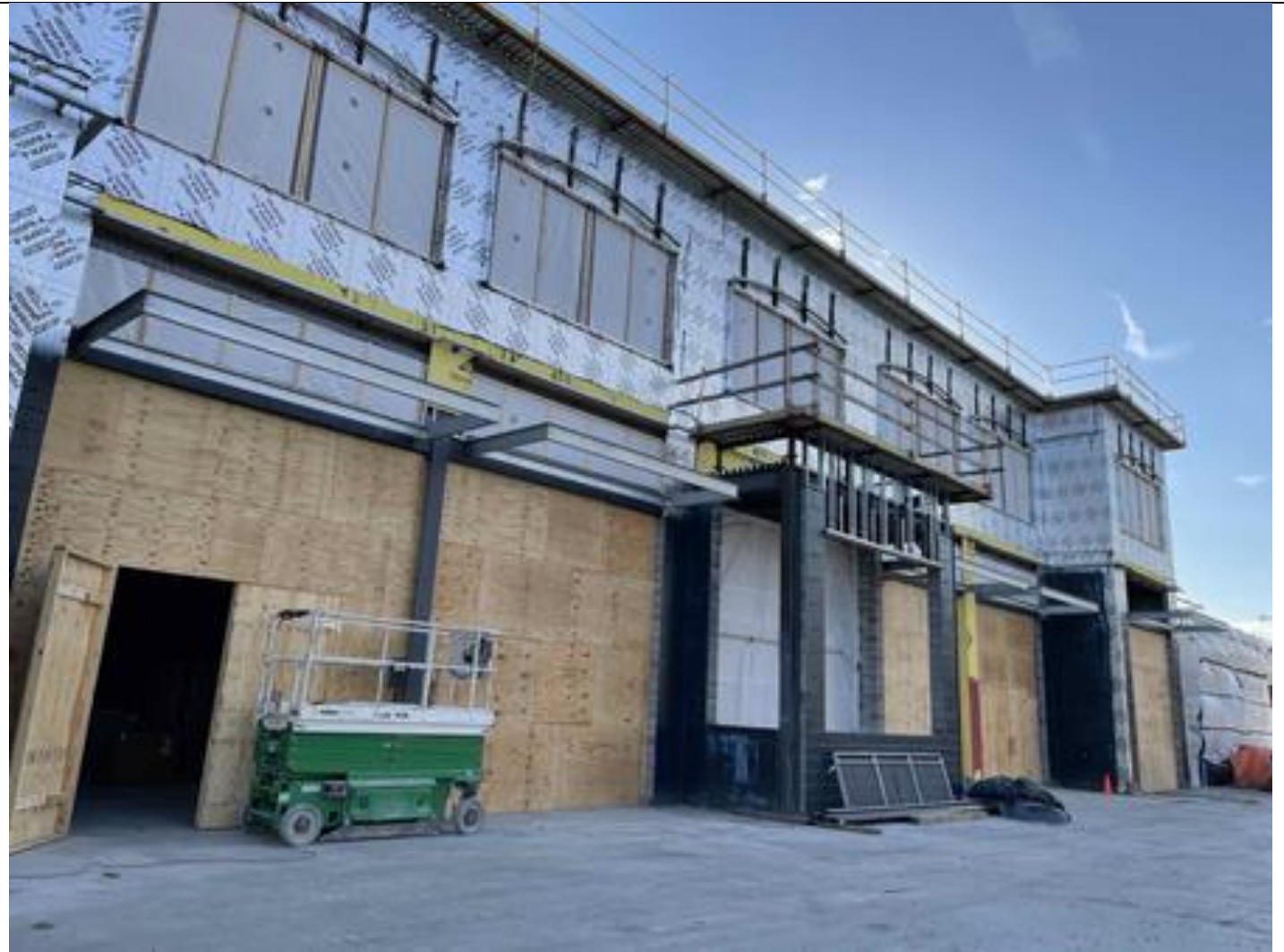
Temporary Overhead Door Installation/AVB Continuing
