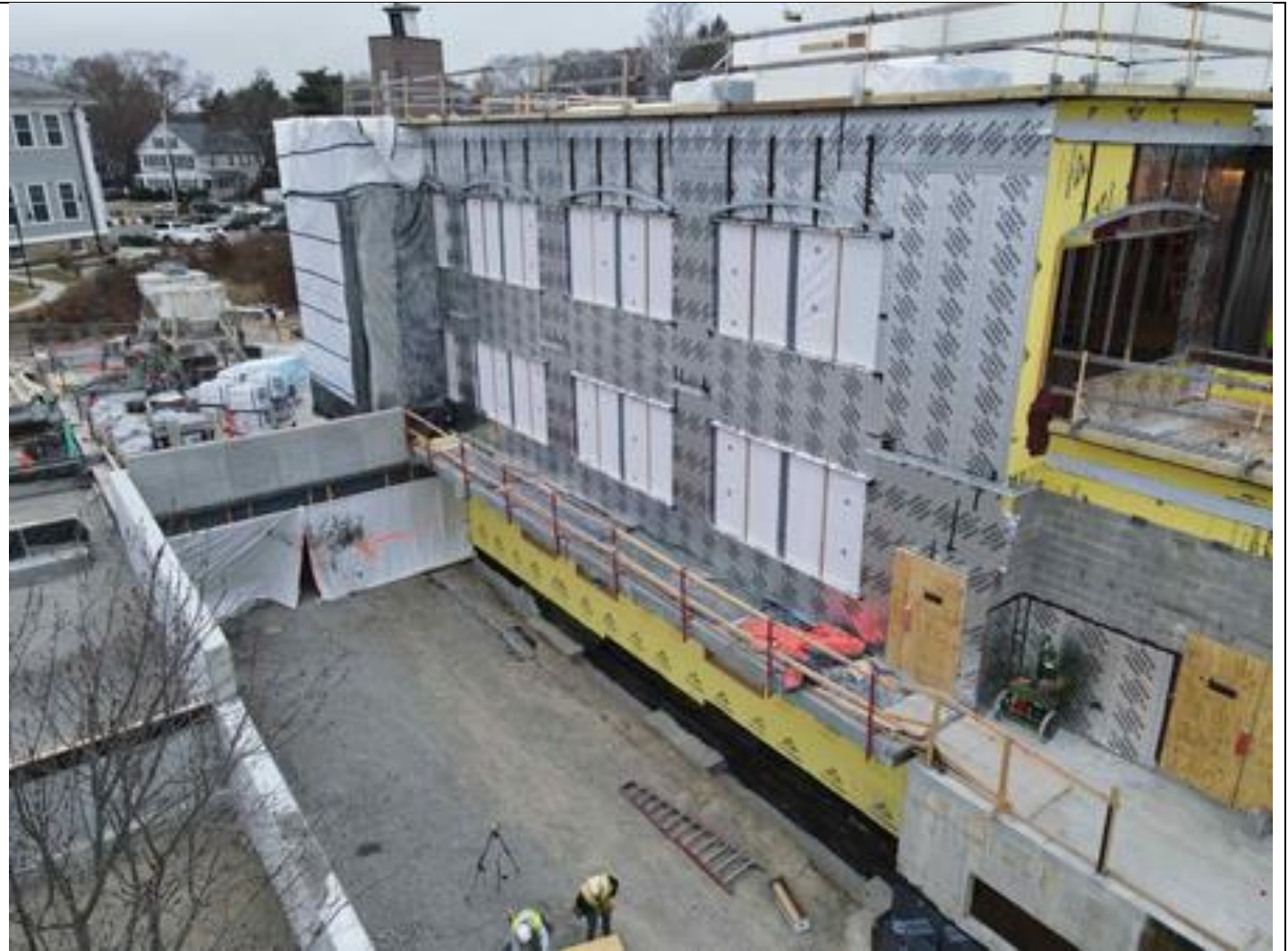
Installation of VR AIB @ Police South Elevation
