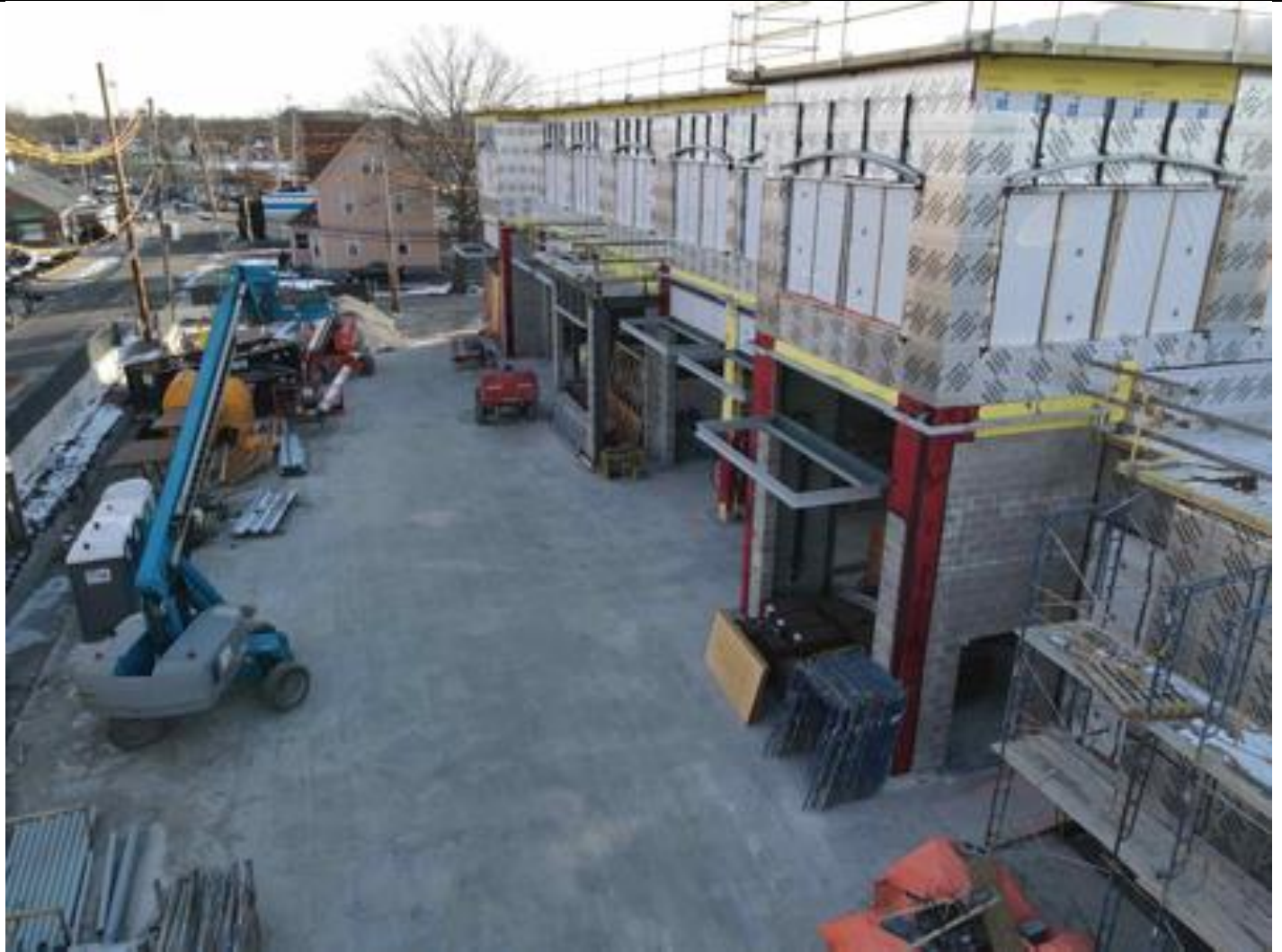
North Elevation Air Barrier System
