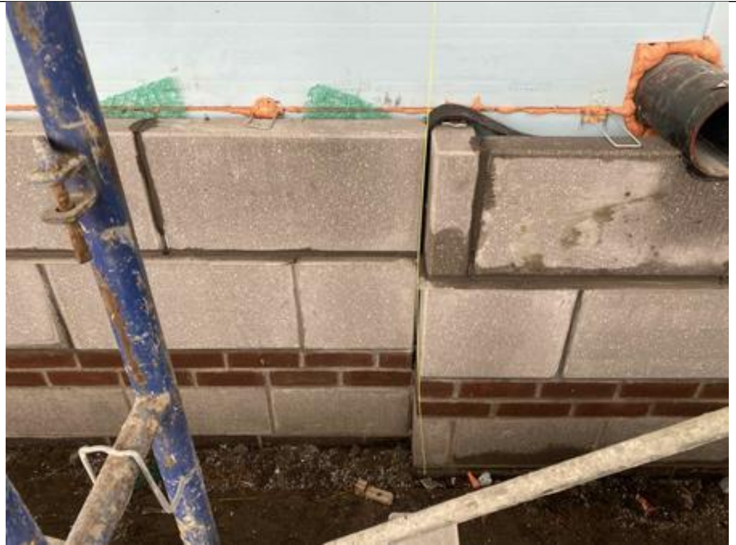
Exterior Masonry "Mock-Up"
