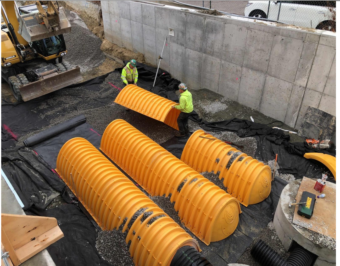
Installation of Subsurface Stormwater Chamber Infiltration System
