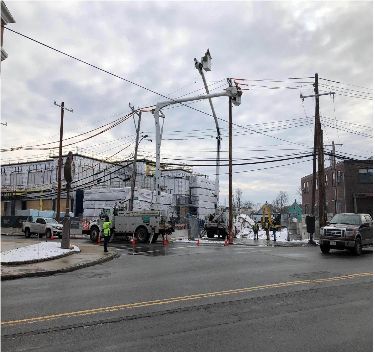
Eversource Line Transfer Crew Relocating OHW
