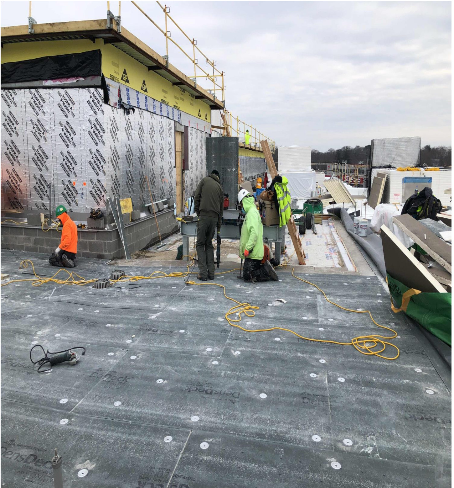
Roofers Installing Police Low Roof
