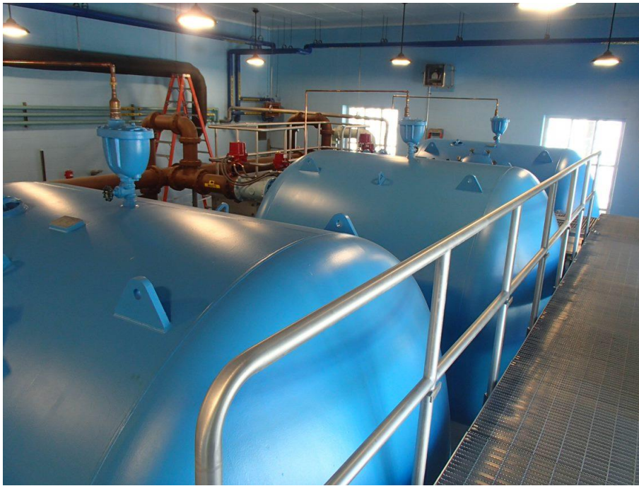
Caption: DWWD New Water Filters Bridge Street Treatment Plant Modernization project
