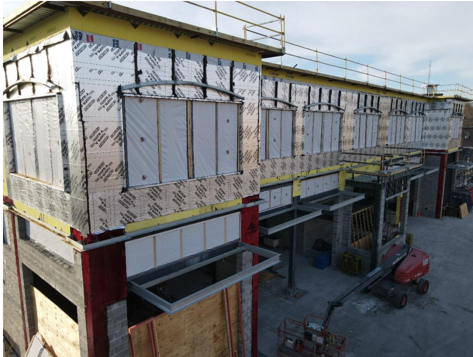
Caption: Photo of exterior walls of the building using a drone on January 13, 2022. The silver material lining the exterior walls is the air and vapor barrier material, designed to prevent the permeation of water vapor.
