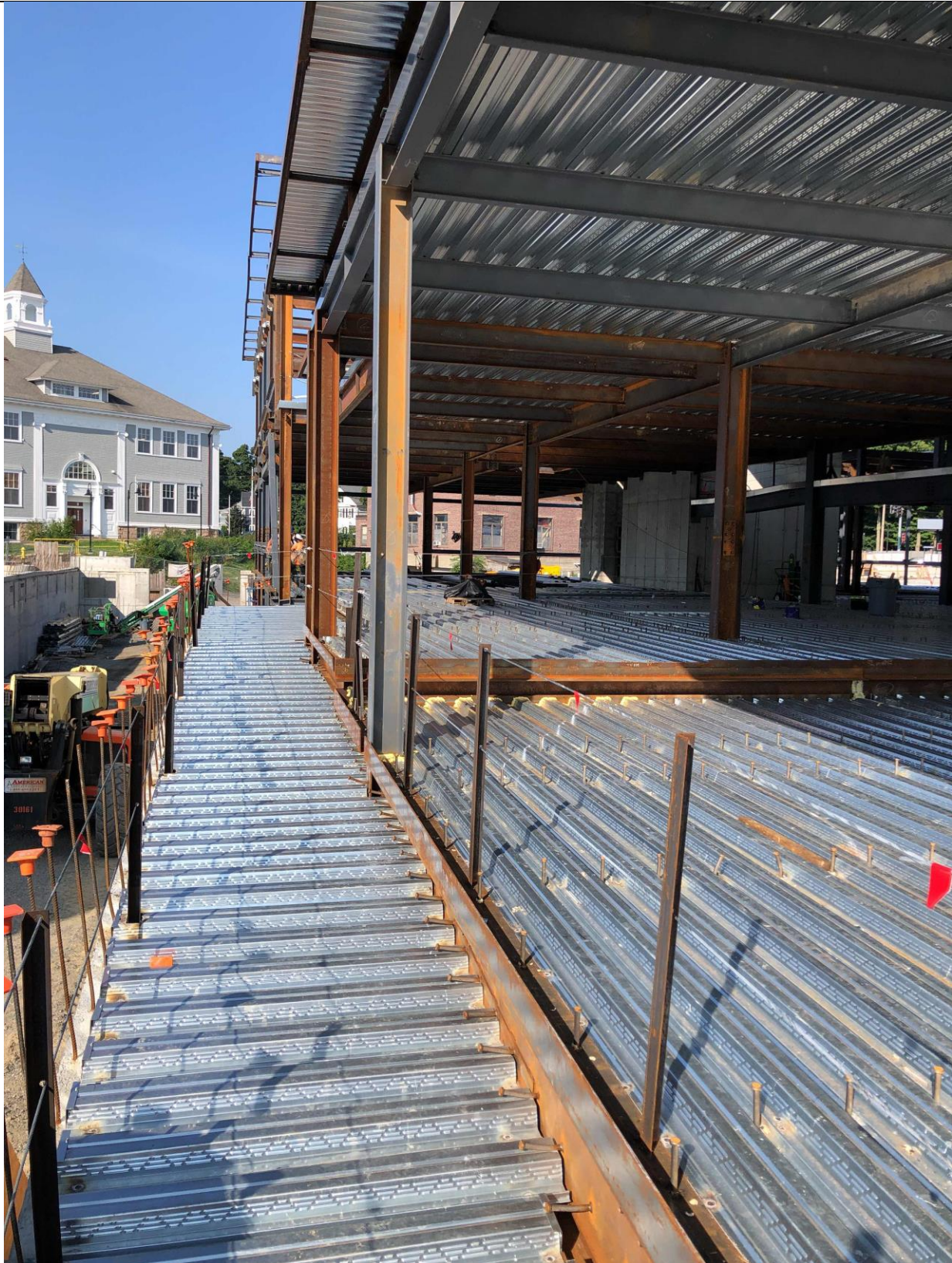
First Floor Structural Steel Decking
