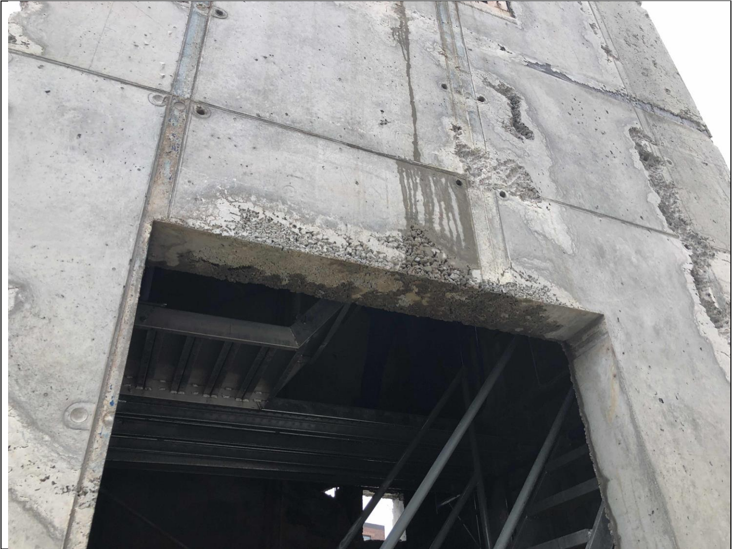
Elevator Shaft Wall Repair
