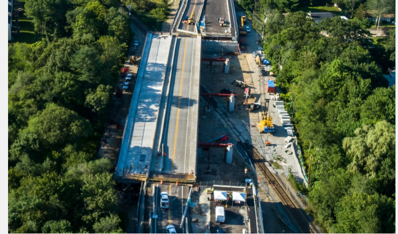
Rt. 18 over Kingston Line in Weymouth – lateral slide
