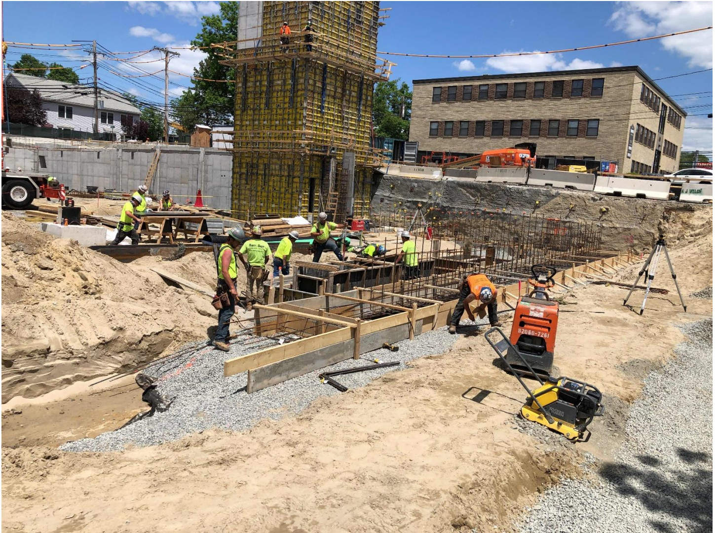
Footing formwork for inside ramp wall - Level 0.
