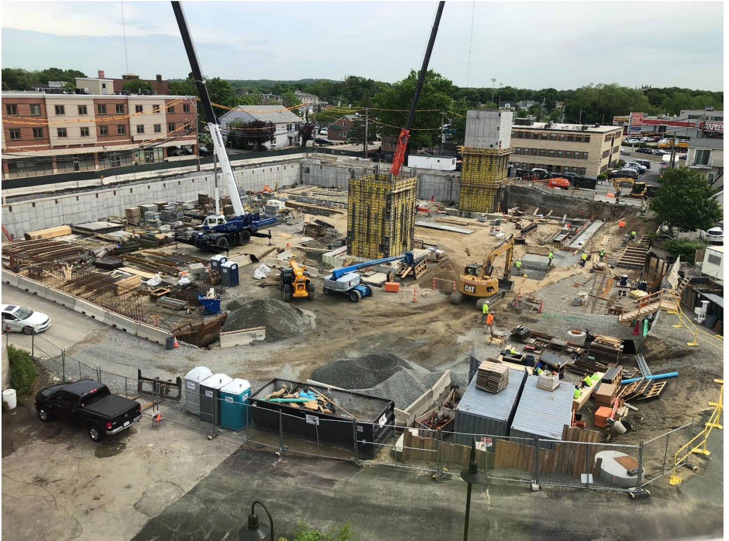
Foundation status as of 5/31/21
