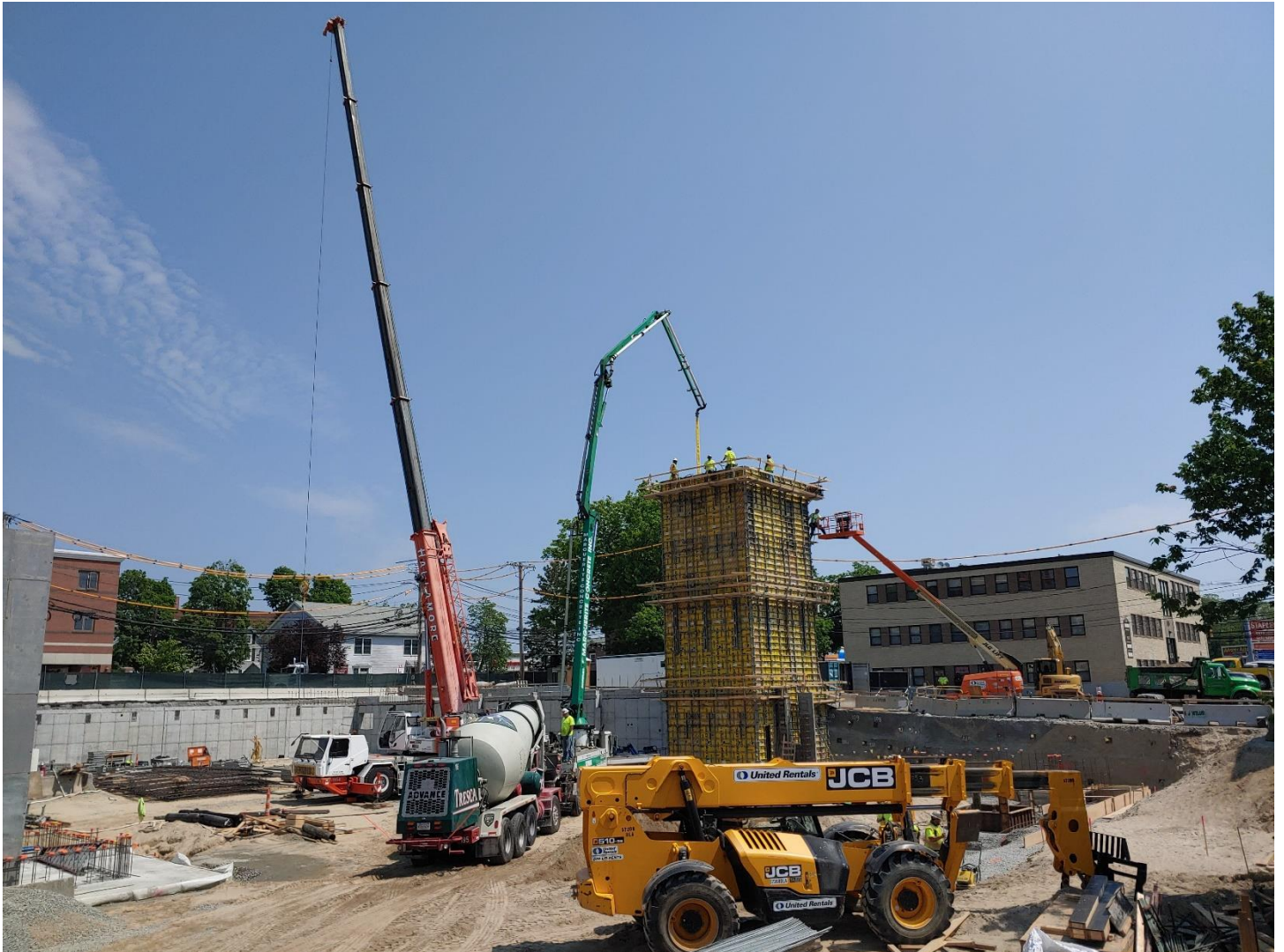
Concrete placement at Stair 2 core tower.
