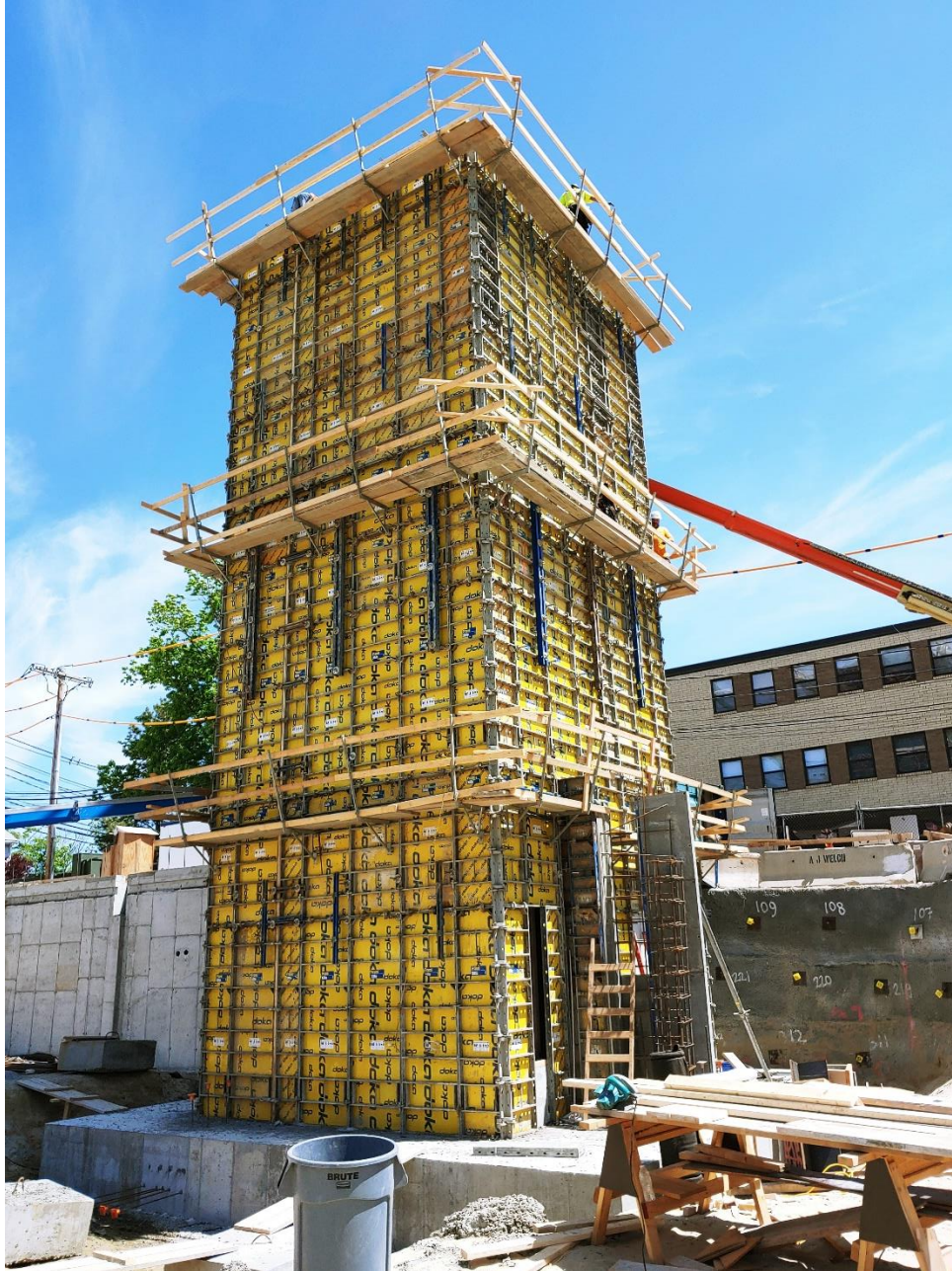
Stair 2 Core Tower formwork.
