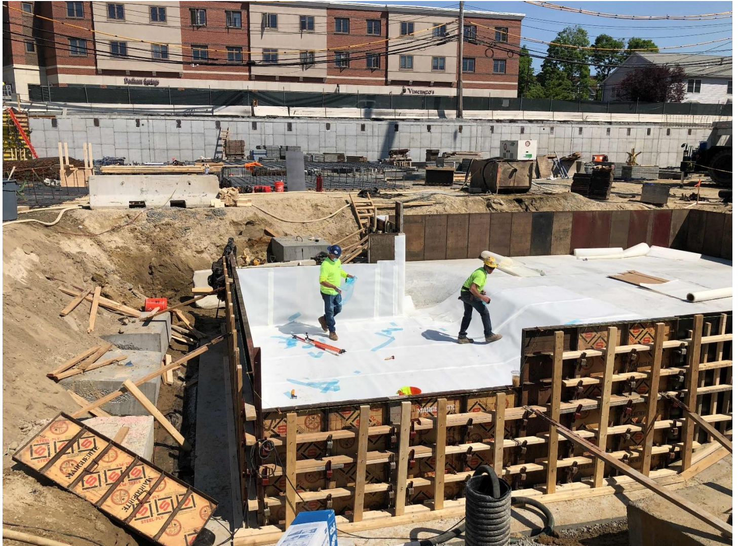
Waterproofing at the bottom of Stair 1 and Elevator towers.
