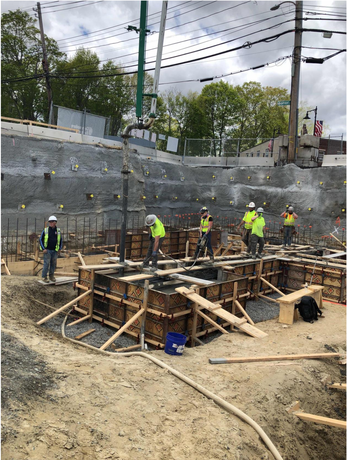
Formwork for foundation footings
