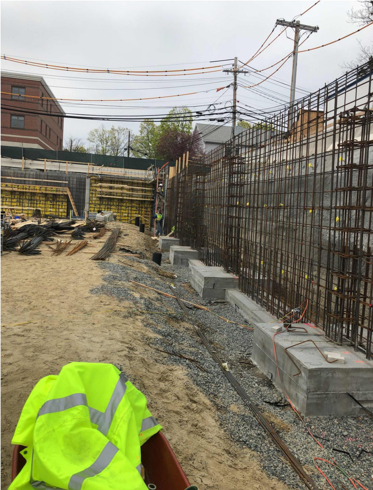
Re-bar for Garage North Wall
