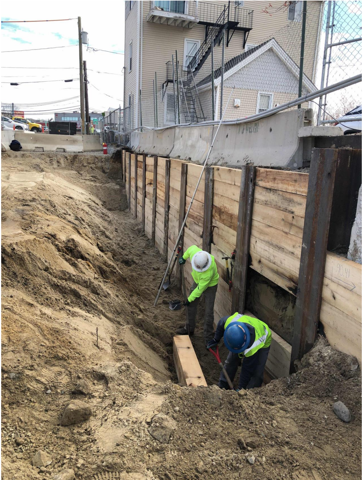
Support of Excavation (SOE) at southern boundary
