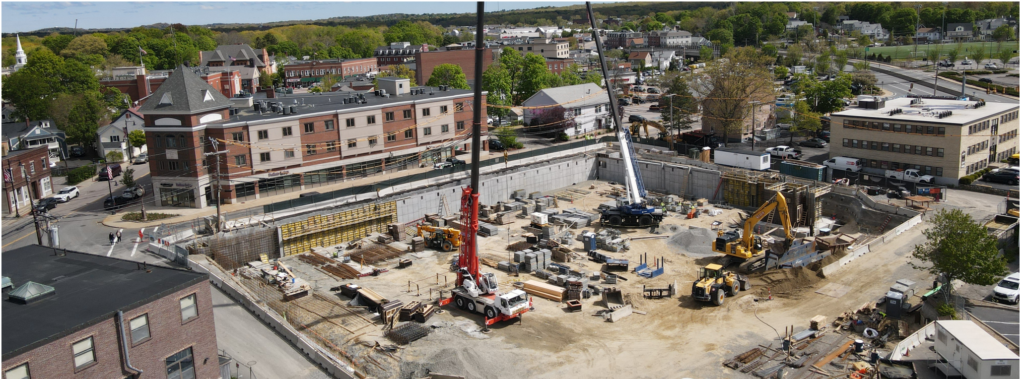
Drone Photos taken on May 12, 2021, provided by Commodore Builders
