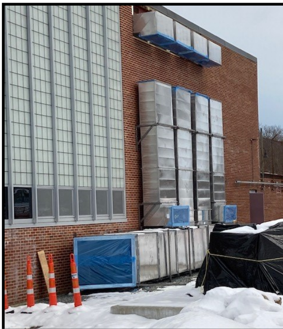
1. New exterior ductwork mains being installed
