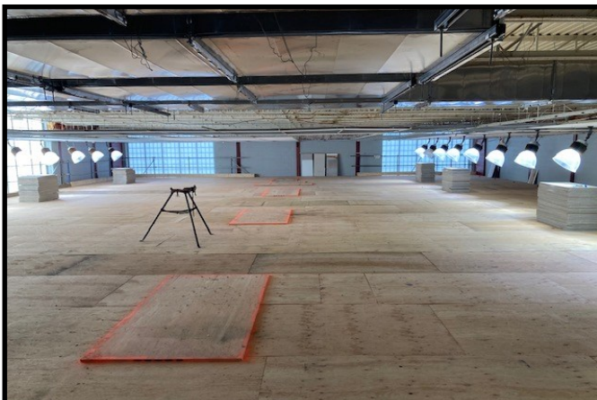
3. View of platform above scaffolding
