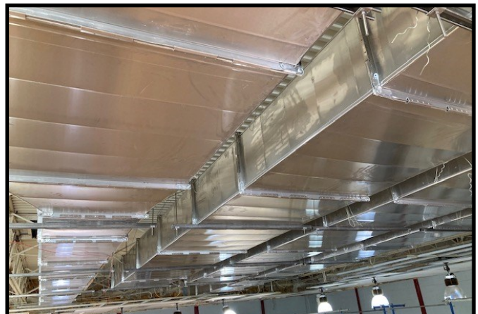
4. New mains being installed inside Pool Building
