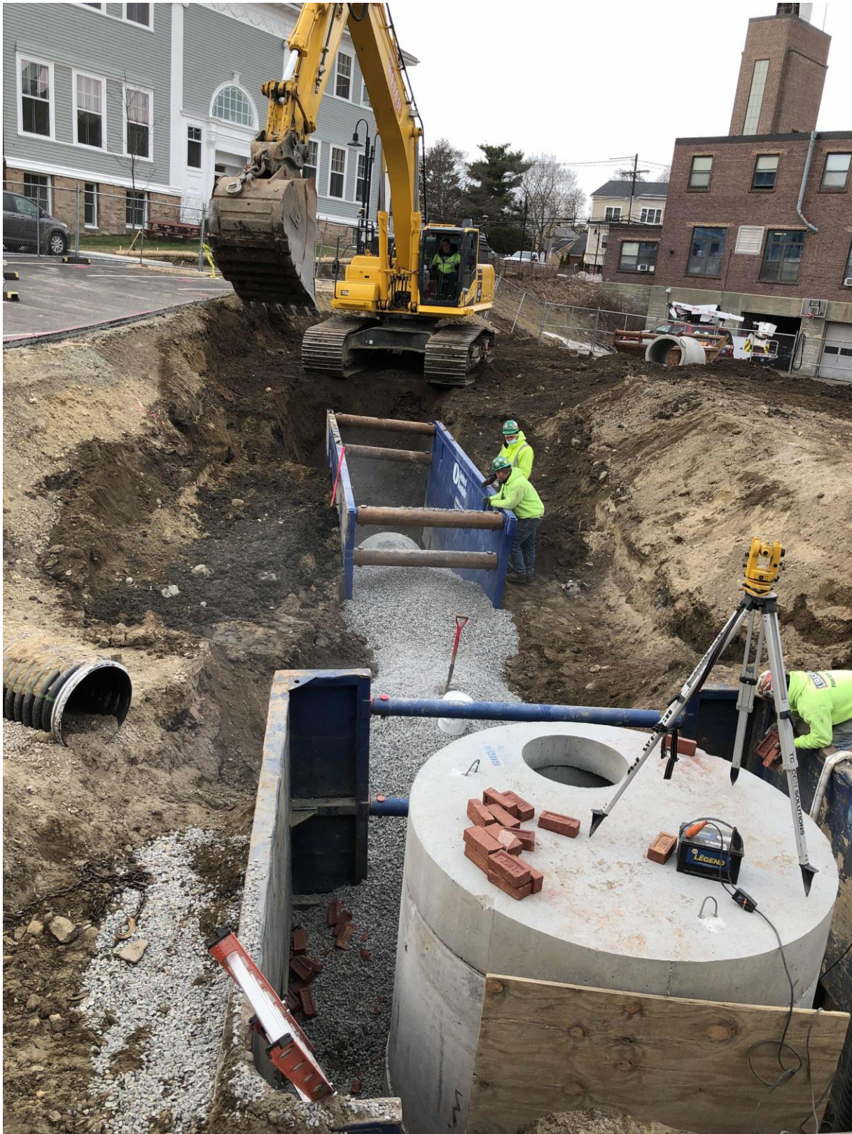
Site drainage install
