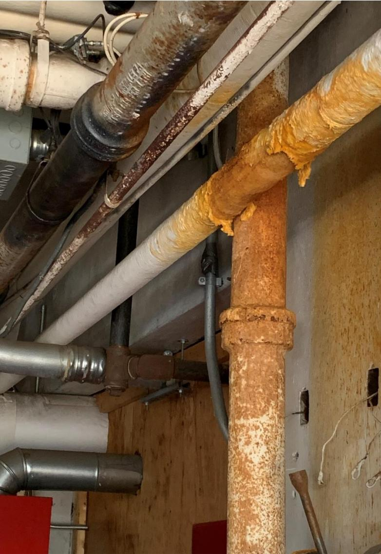
Deteriorated drainage pipes
