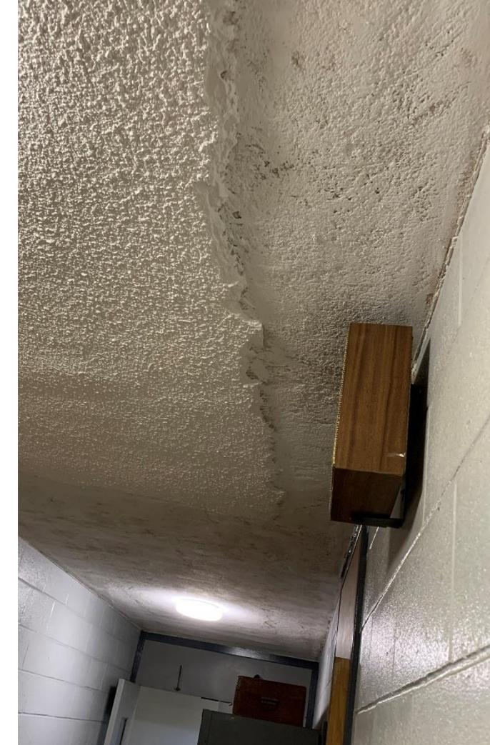
Deteriorating ceiling with material partially removed due to water damage and asbestos content.
