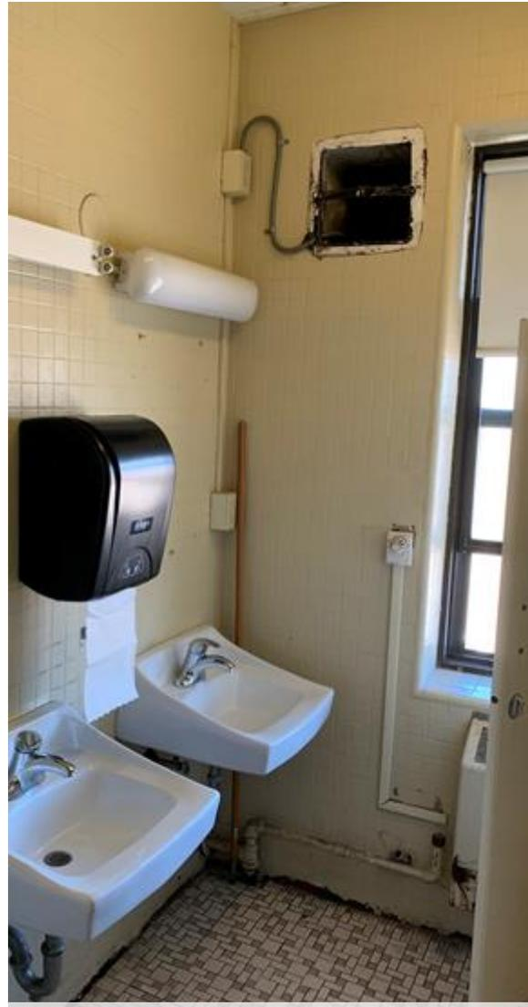
Restrooms are not code compliant and are not properly ventilated
