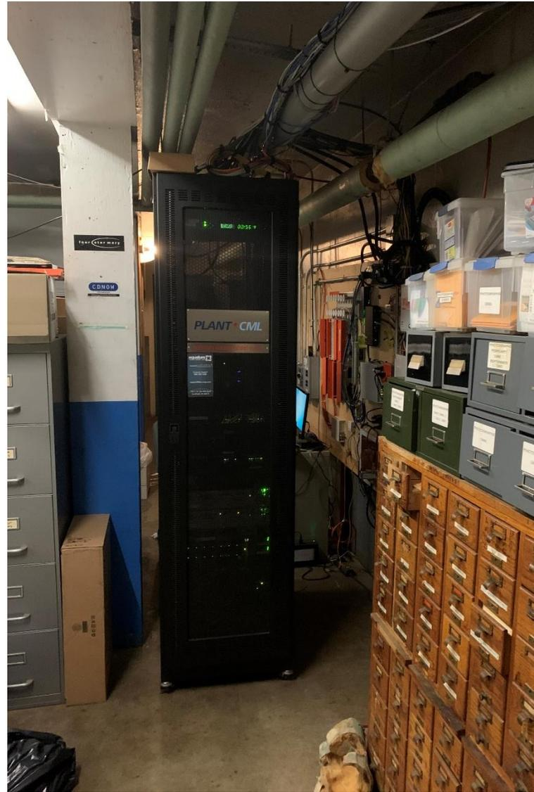
911 System Located in Storage Room with no HVAC
