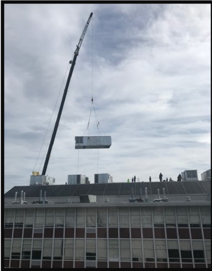
Veterans Development Corp. of Norwell lifting one of three 40+ ton rooftop units
