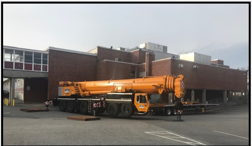
Liebherr LTM1300 Crane weighing over 700,000 lbs. by Astro Crane of Boxborough
