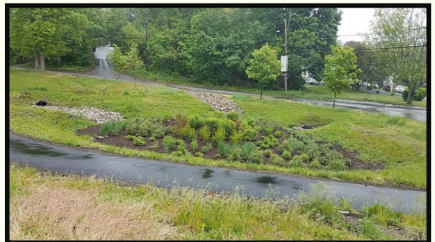
Colburn Street Bioretention Basin
