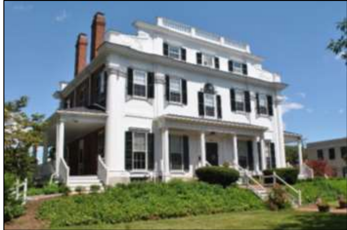
Figure 5.3 – Dedham Community House
